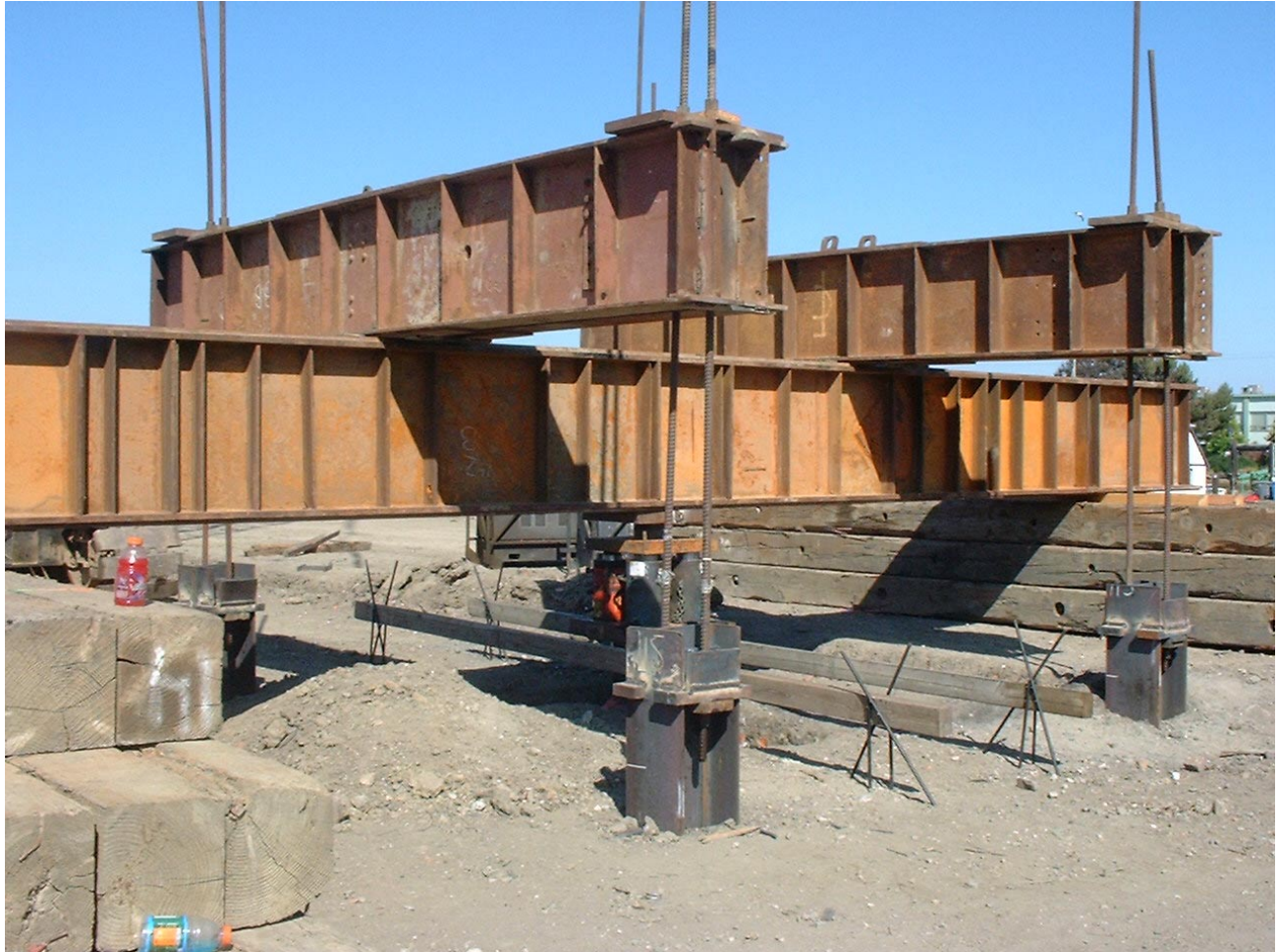
Frame during 1040-kip load test.
