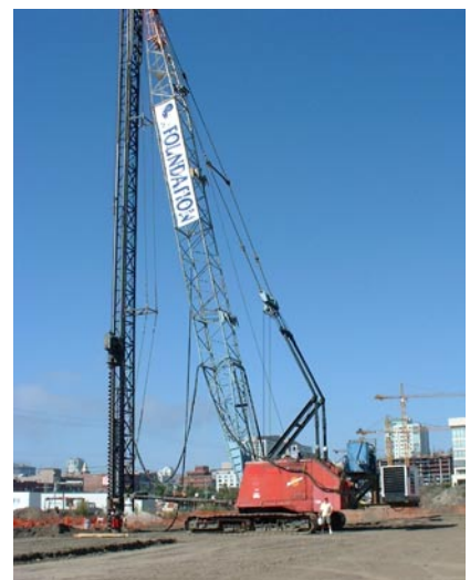
Installation of foundation piles.
