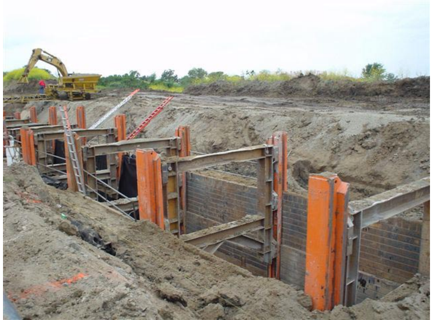
Sewer line trench shoring system.
