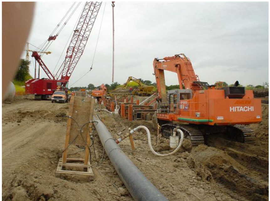
Excavation for gravity sewer line.
