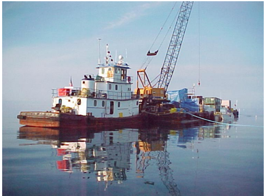
Crane barge installing reef restoration modules at operation site.
