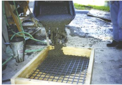
Template for pre-installation of drilled shafts.
