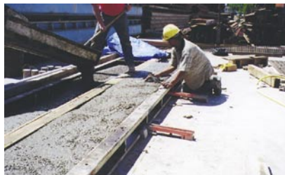
Template for pre-installation of drilled shafts.
