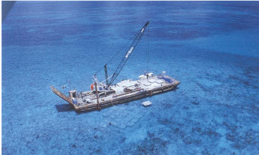
Lowering of pre-cast concrete panels.
