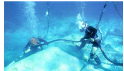
Placement of pre-cast concrete panels.
