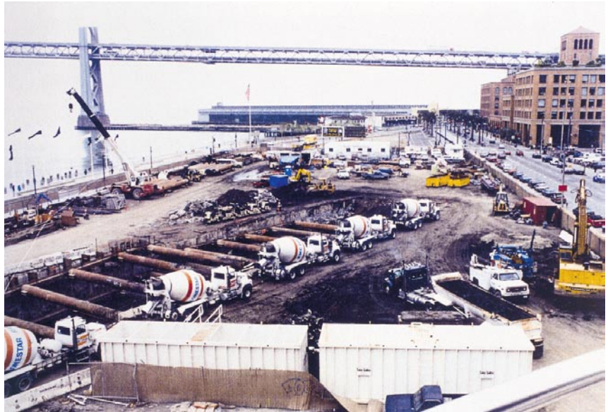
Excavations shared using "soldier piles and tremie concrete" (SPTC) Method.
