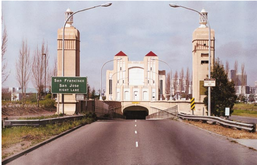
Alameda approach to the Posey Tunnel.
