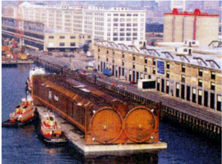
Tunnel segments being shipped by barge.
