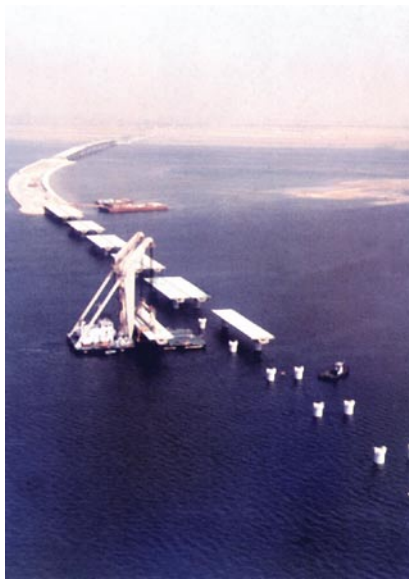
Placement of deck panels.
