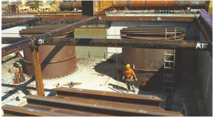
Installation of large-diameter steel piles for the new Carquinez Bridge, CA.
