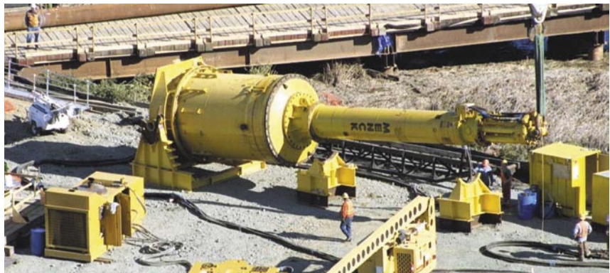
Hammer for installation of large-diameter test casings for the Benicia-Martinez Bridge.
