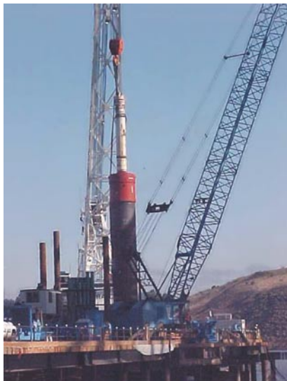
Large-diameter pile installation for the Benicia-Martinez Bridge, CA.
