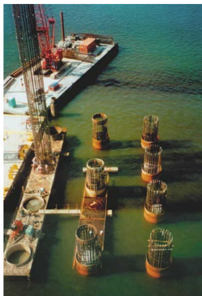
Drilled shafts for the mid-river main bridge piers.
