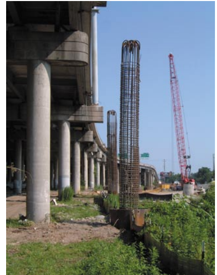
Drilled shafts for the high level approach piers.
