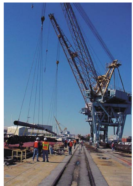
Load-out of drilled shaft rebar cages.
