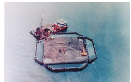
Construction of caisson-encased Tarsuit Island.
