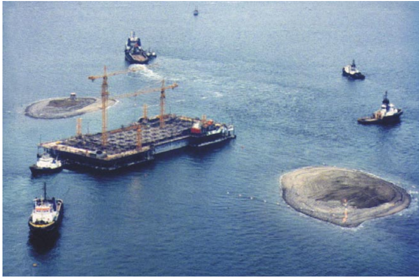
Positioning of Great Belt East Bridge Caisson.
