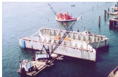
Float-in and set-down of 5,400 ton concrete caissons for Tarsuit Island.
