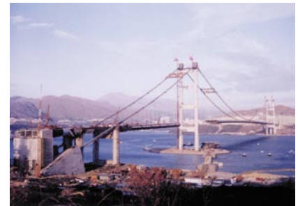
Tsing Ma Bridge nearing completion.
