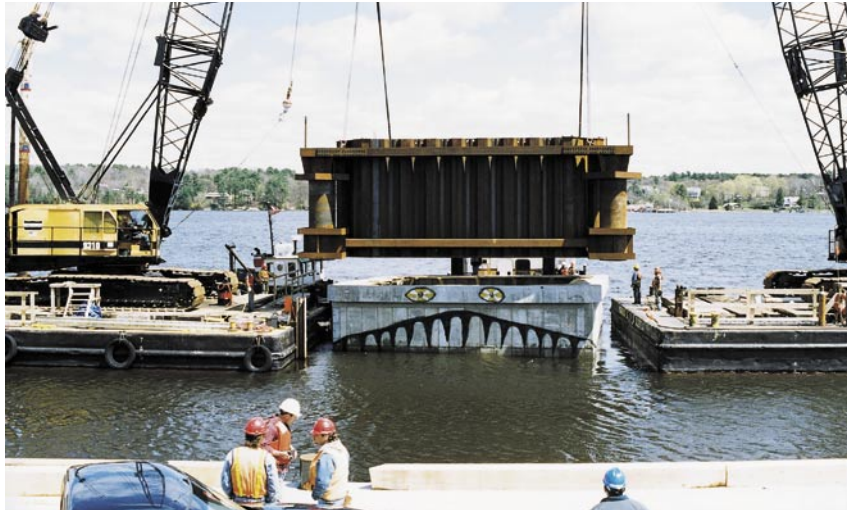
Mating of follower cofferdam to floating precast footing shell.
