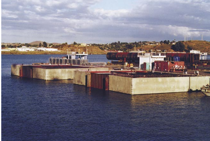
Float-in cofferdams at dock side.
