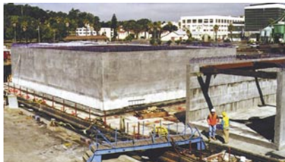
Interior of completed float-in cofferdam.
