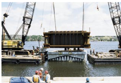
Design-build of foundations for the Bath-Woolwich Bridge, ME.
