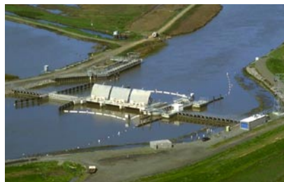
Salinity control structure, Suisun Bay, CA.
