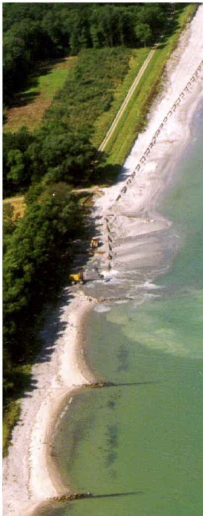
Large-scale beach nourishment by pipeline.
