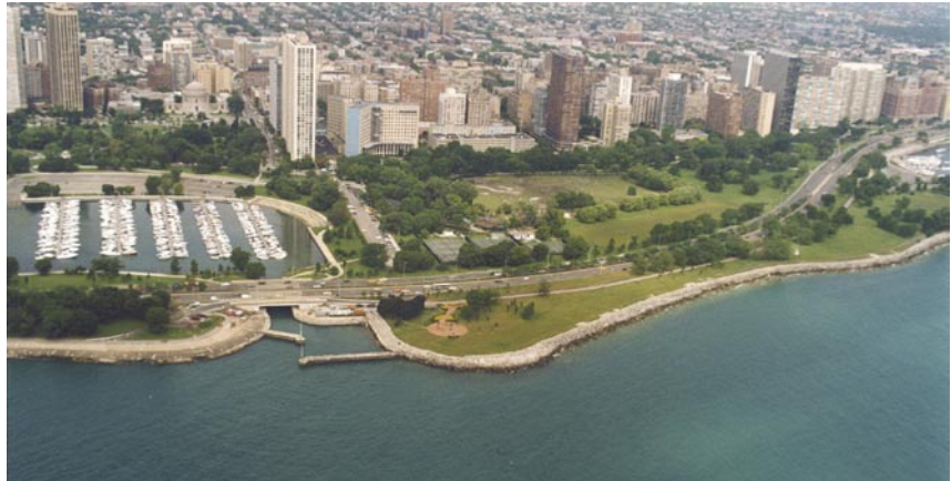
Storm damage reduction project, Chicago shoreline, Lake Michigan, IL.
