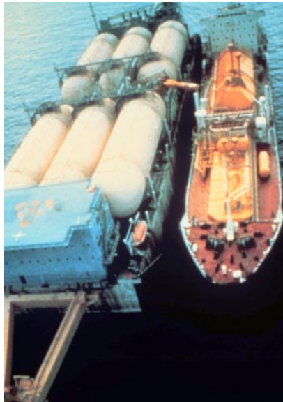
Sakti Ardjuna concrete floating terminal.
