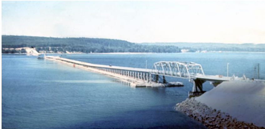
Evergreen Point floating bridge.
