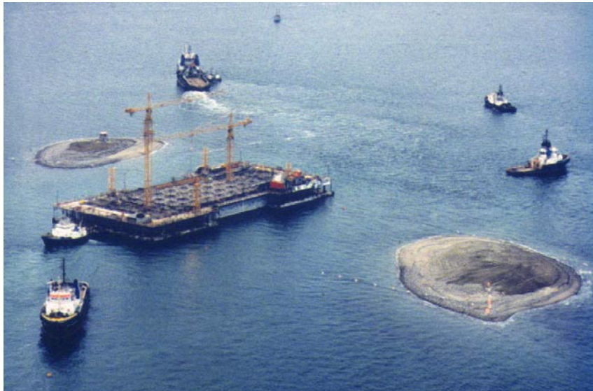
Positioning of Great Belt East Bridge Caisson.
