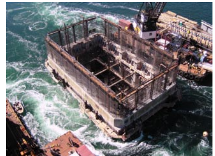
Tacoma Narrows Bridge main pier caissons.
