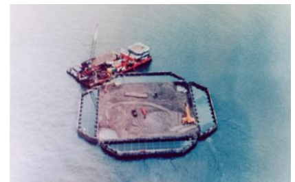
Construction of caisson-encased Tarsuit Island.
