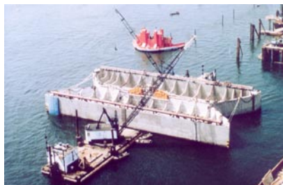
Float-in and set-down of 5,400 ton concrete caissons for Tarsuit Island.
