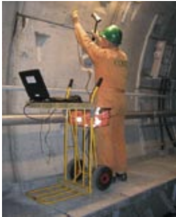
Tunnel wall testing.
