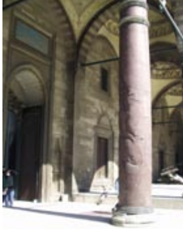
Red sandstone column in Istanbul with cracks due to low bending-tensile strength.
