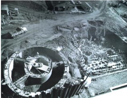
Foundations for Nuclear Power Plant Humboldt Power Station, California.
