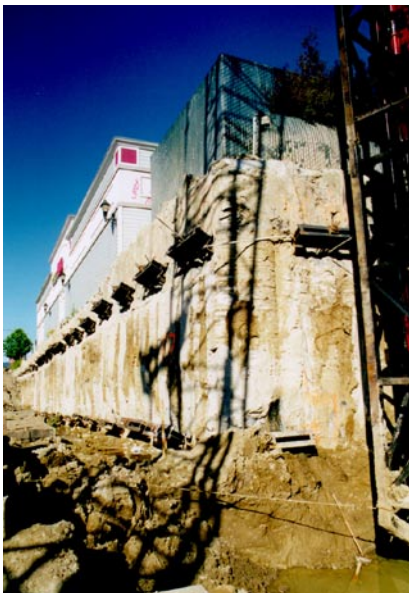
Soil Mix Wall.
