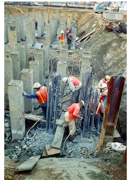
Header pipe. Ala Moana, Hawaii.
