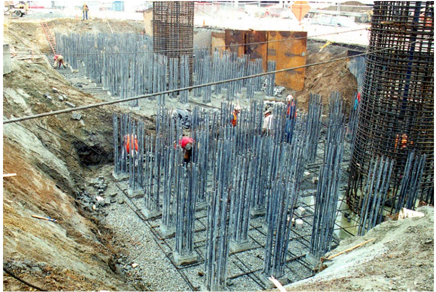
Parking structure pile foundation. San Francisco International Airport.
