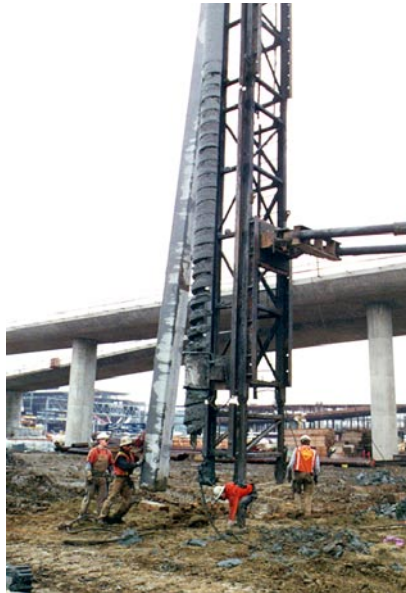
Cushion preset in pile hammer. Ala Moana, Hawaii.
