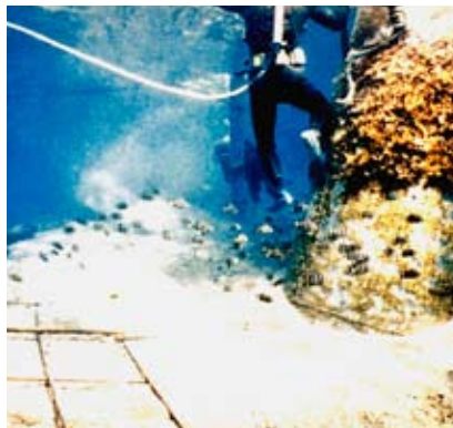
Placement of high quality underwater concrete
