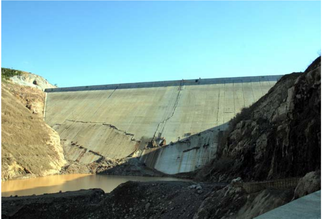
Inspection of concrete cracks in dam
