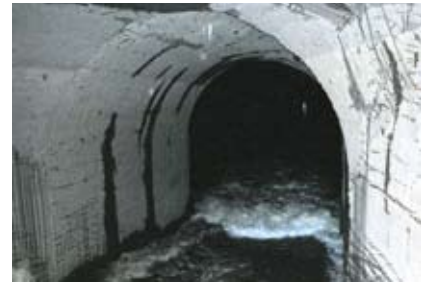
Inspection of damage in concrete diversion tunnel
