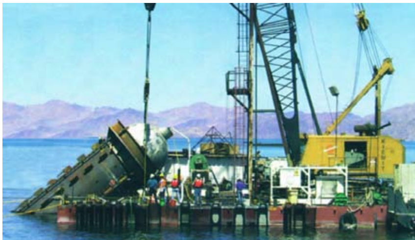
Installation of Lake Mead water intake structure
