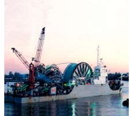
Pipelaying vessel installing 3,700 ft lengths of pipe
