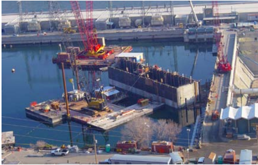
Float-in of fish bypass structure for Rocky Reach Dam
