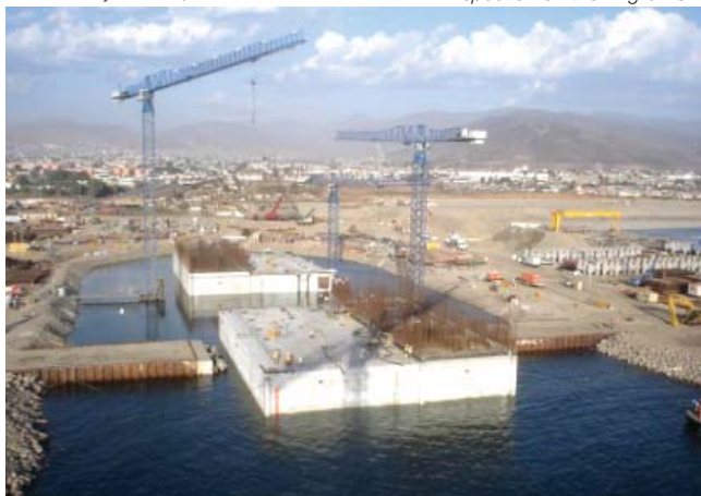
Float out of concrete segment
