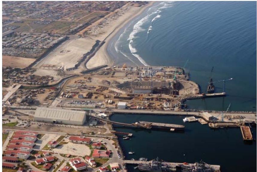
Casting Basin for the construction of Breakwater Caissons, Ensenada, Baja California
