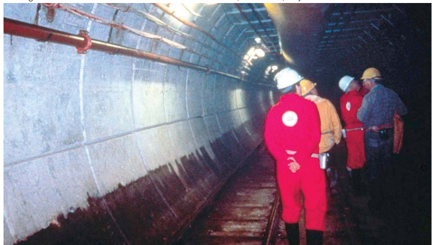
Inspection of the English Channel Tunnel
