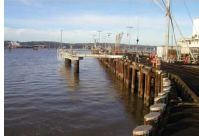
Tesoro Terminal MOTEMS Inspection
