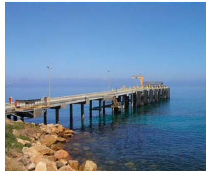
New US Navy Pier, San Clemente Island, CA.
