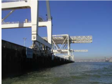
Port of Oakland Berth 35-37, CA
